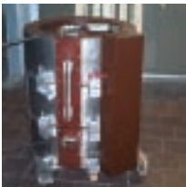
7 50 Hz filter used for reducing induced EMI in 3 KVcc railway lines
